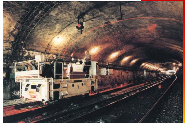
Inspection vehicle for subway
